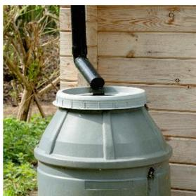
A rainwater tank is a water tank used to collect and store rainwater runoff, typically from rooftops via pipes. Rainwater tanks are devices for collecting and maintaining harvested rain. A rainwater catchment or collection system can yield 2,358 litres of water from 2.54 cm of rain on a 92.9 m<sup>2</sup> roof. This water can then be used for watering your lawn, gardens and house plants; cleaning off gardening tools; and even washing your car.
